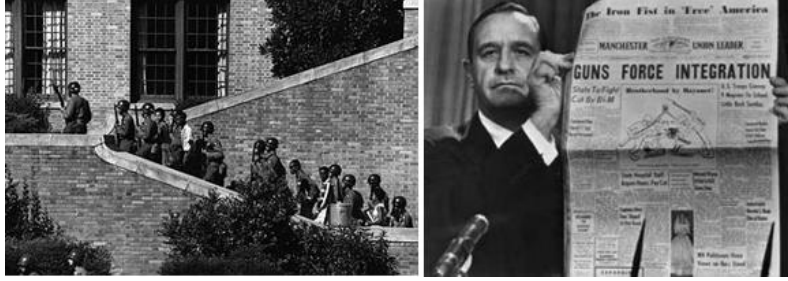
The "Little Rock Nine" are escorted inside Little Rock Central High School by troops of the 101st Airborne Division of the United States Army.
